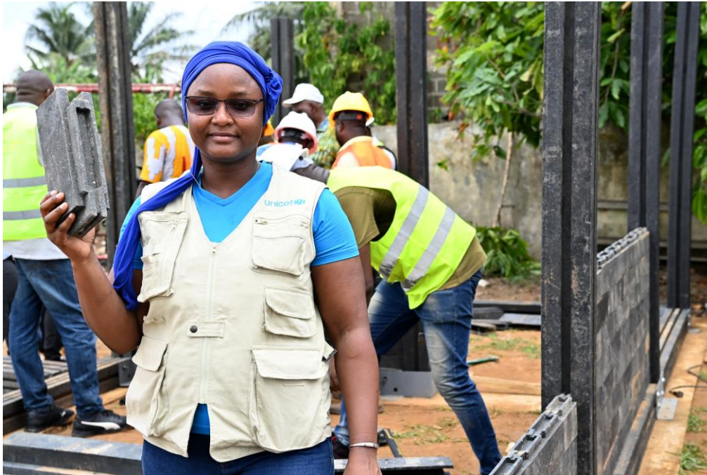
A UNICEF employee holding up a plastic brick at a construction site. © UNICEF/Dejongh
